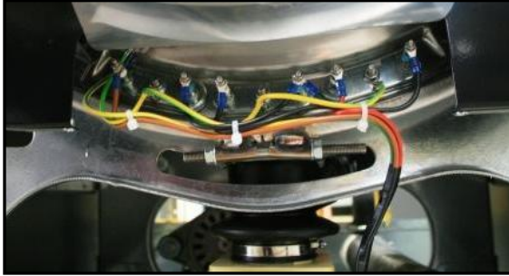
Heating elements in the front
